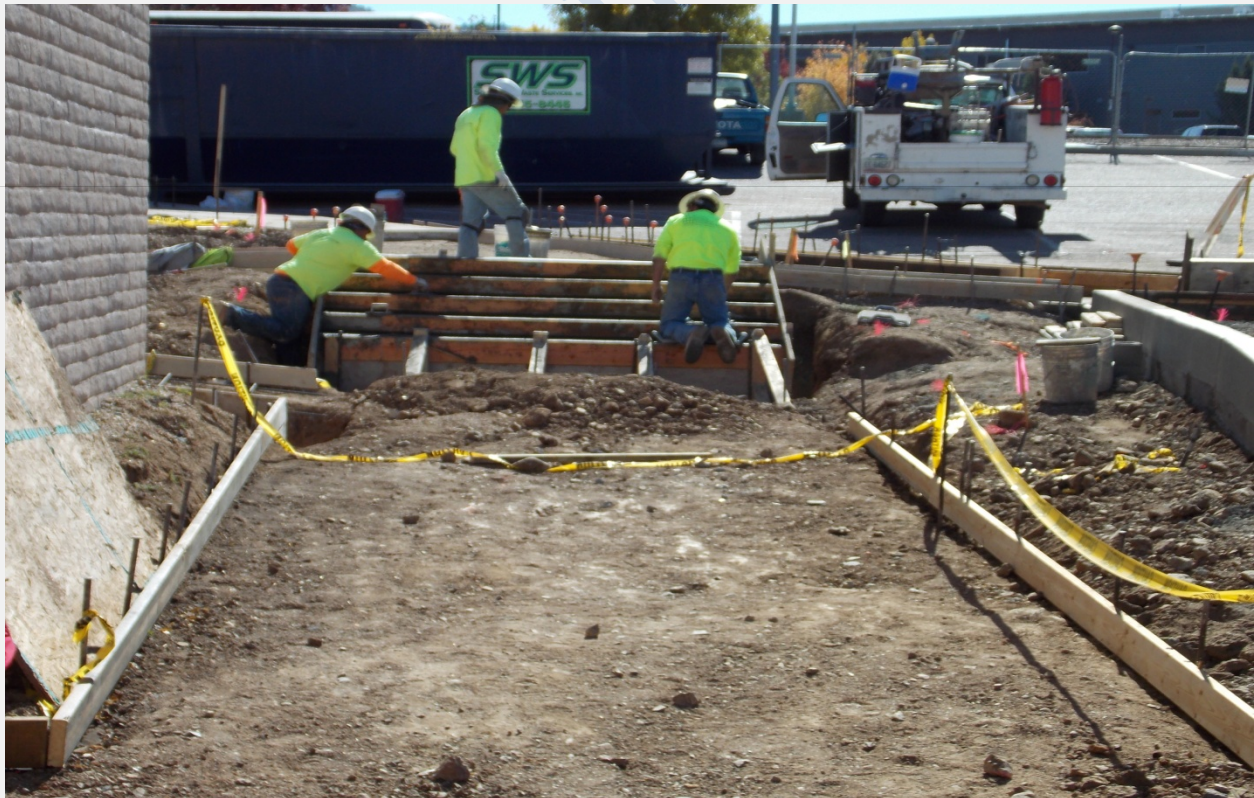
New Walkway Construction on West side of Marapai
