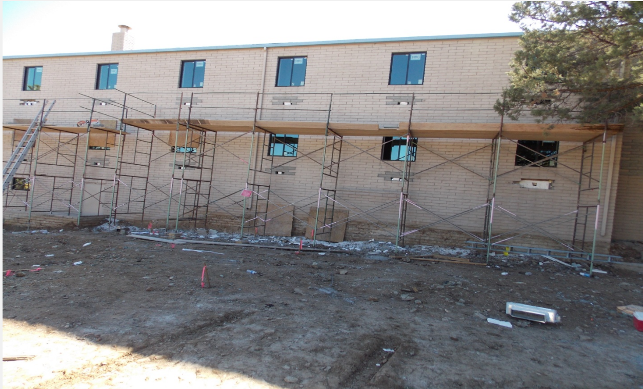
Masonry Work and Installation of New Windows
