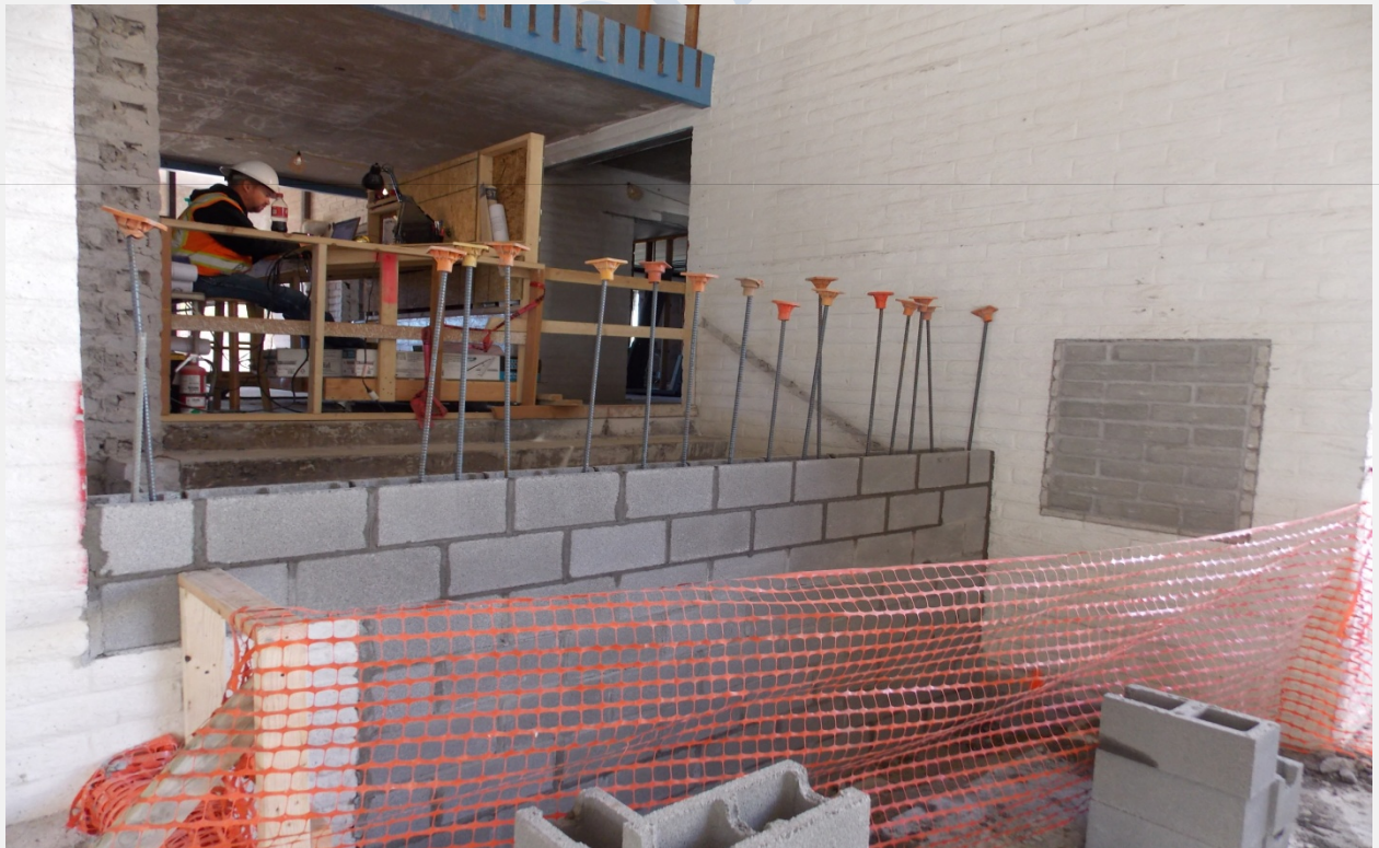
Masonry Work for New Reception Area
