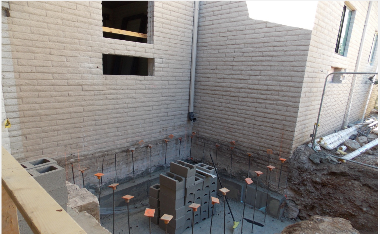
Constructing of Elevator Shaft
