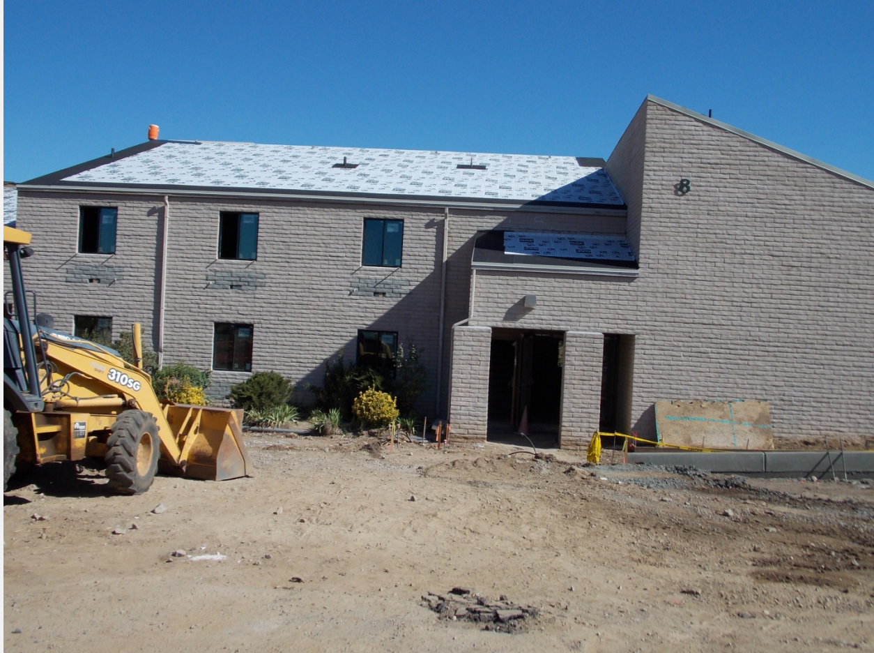
Installation of New Roof
